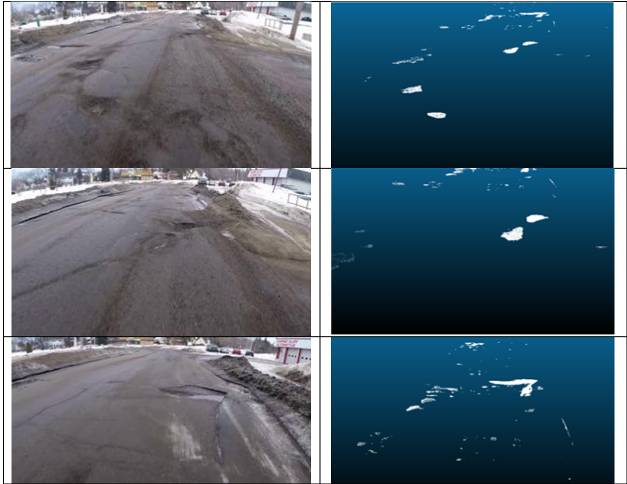
Figure 2: Select frames from the Sudbury.com video (2019) and their matching pothole detection results; from top to bottom, the left images will be referred to as Figure 2a, 2b, and 2c and the right images will be referred to as Figure 2d, 2e, and 2f
